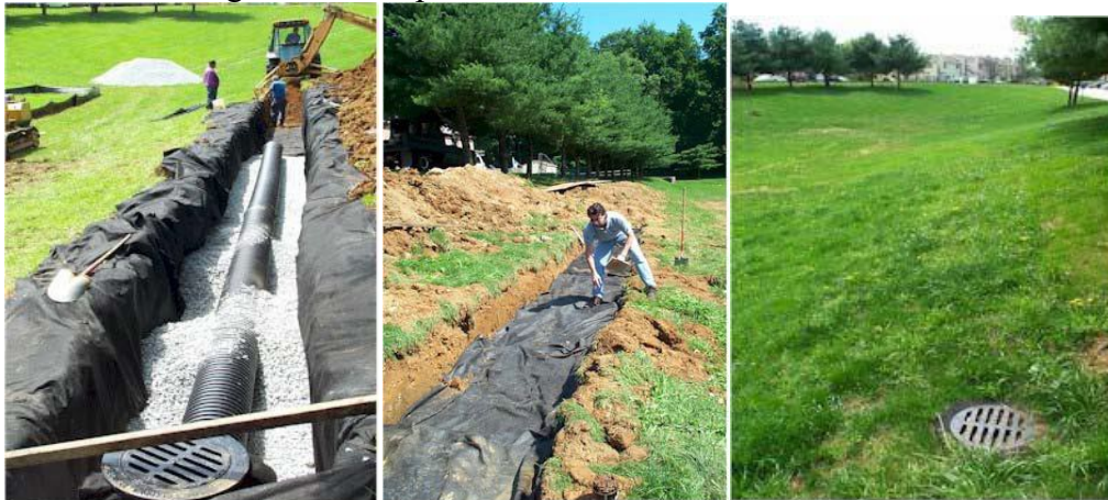
Figure 3: Example of Infiltration Trench Installation
